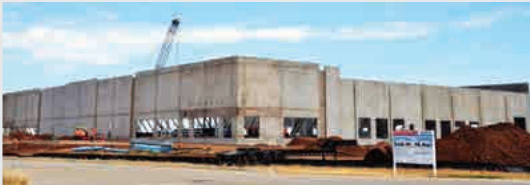
Spec Building Construction Underway
